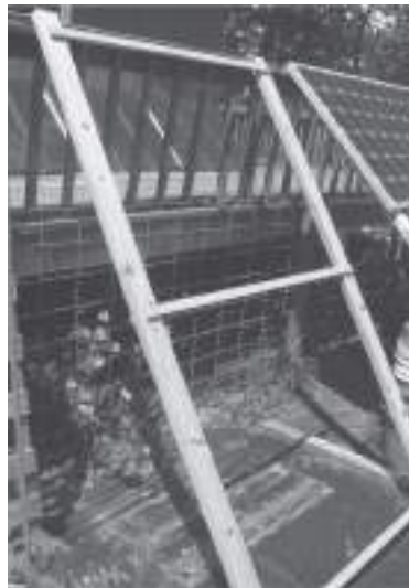
Wooden deck-mounted racking awaiting new panels
